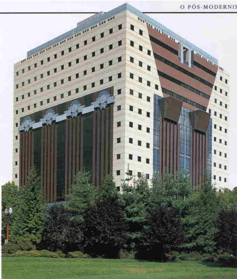
PUBLIC SERVICES BUILDING, PORTLAND, OREGON, 1980-1982
